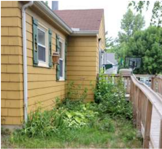
Before the work began
